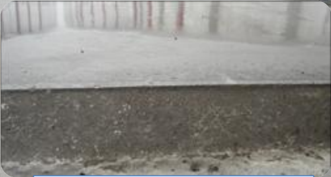
PATCHCRETE layer varies up to 50 mm or 2".
