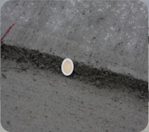
PATCHCRETE layer is thinner than 20 mm or ¾".
